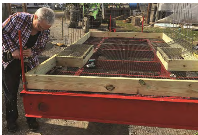
Hannah Smith-Brubaker builds a 2"x6" pressure treated frame on the deck of the trailer.
